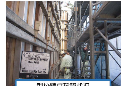
型枠精度確認状況
